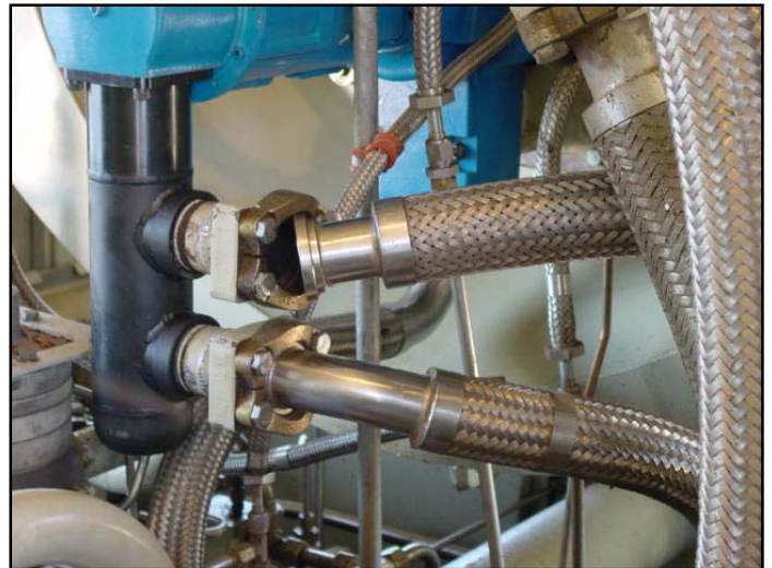
Figure 8. Exhaust Hose Installation
