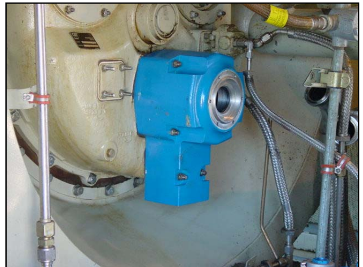
Figure 6. TDI Adapter Installation
